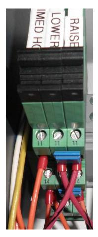
The Meter box wiring connects to the meter box terminal strip in the control box (see image below).
